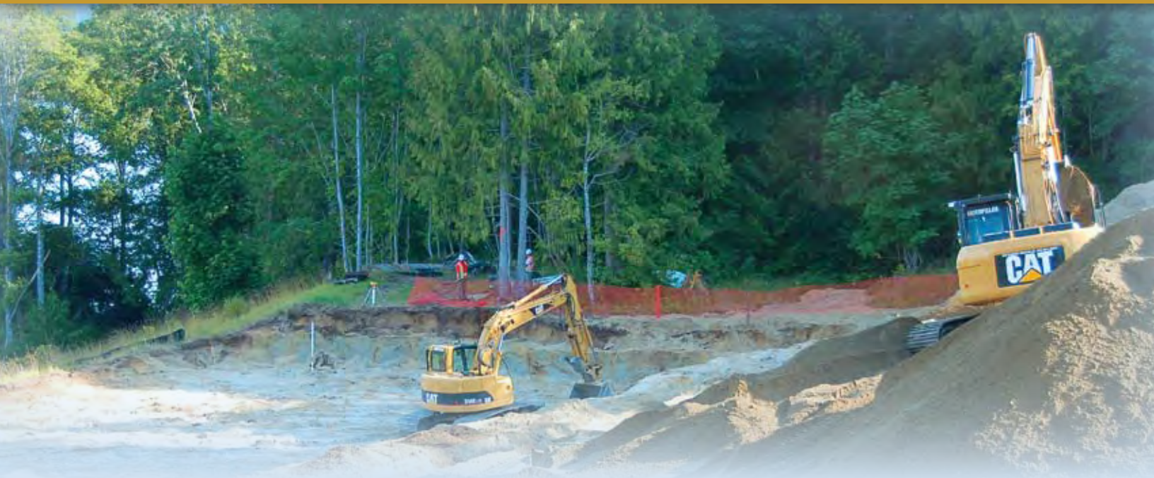
Start of construction for the Vancouver Island University Centre for Shellfish Research, Deep Bay Field Station.
