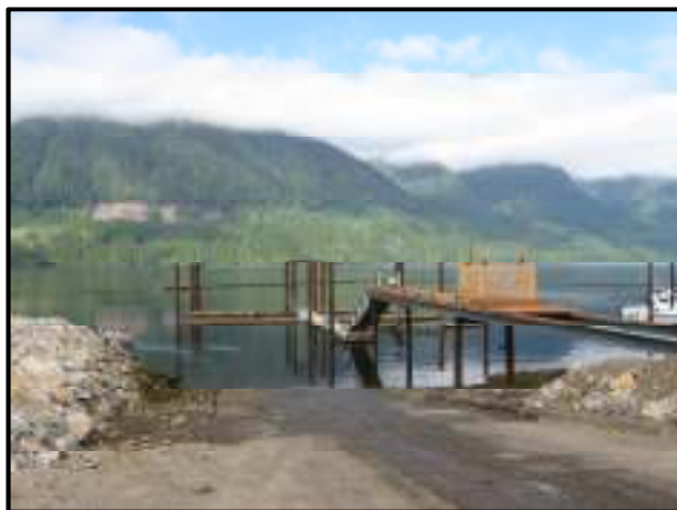
Steel girders on pilings support a 25 m fixed pier.
