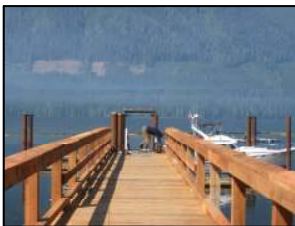
Cedar decking & rails was custom milled locally.
