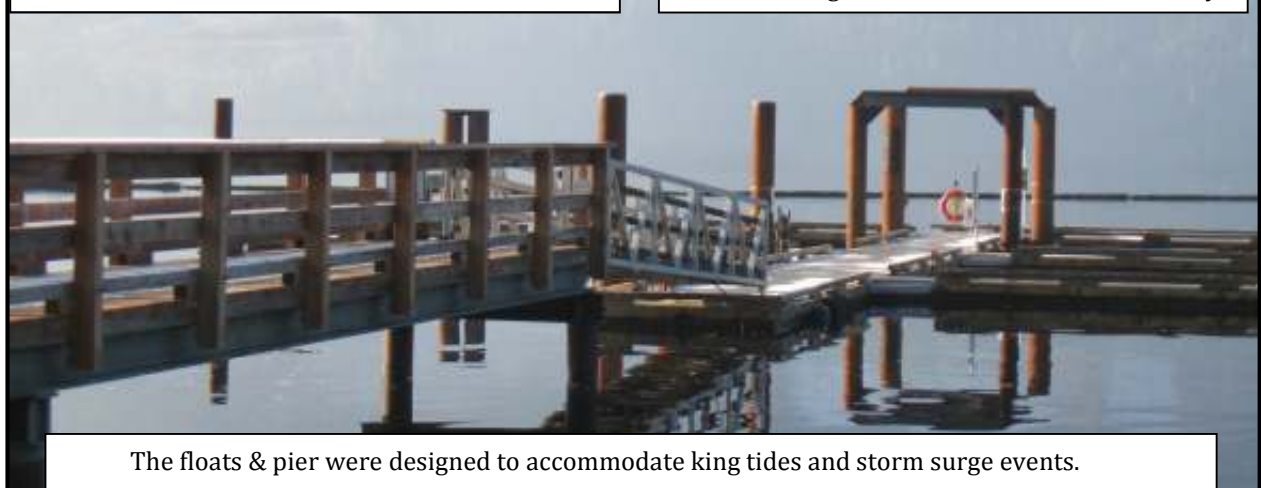
Cedar decking & rails was custom milled locally.
