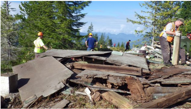
Old structure dismantled
