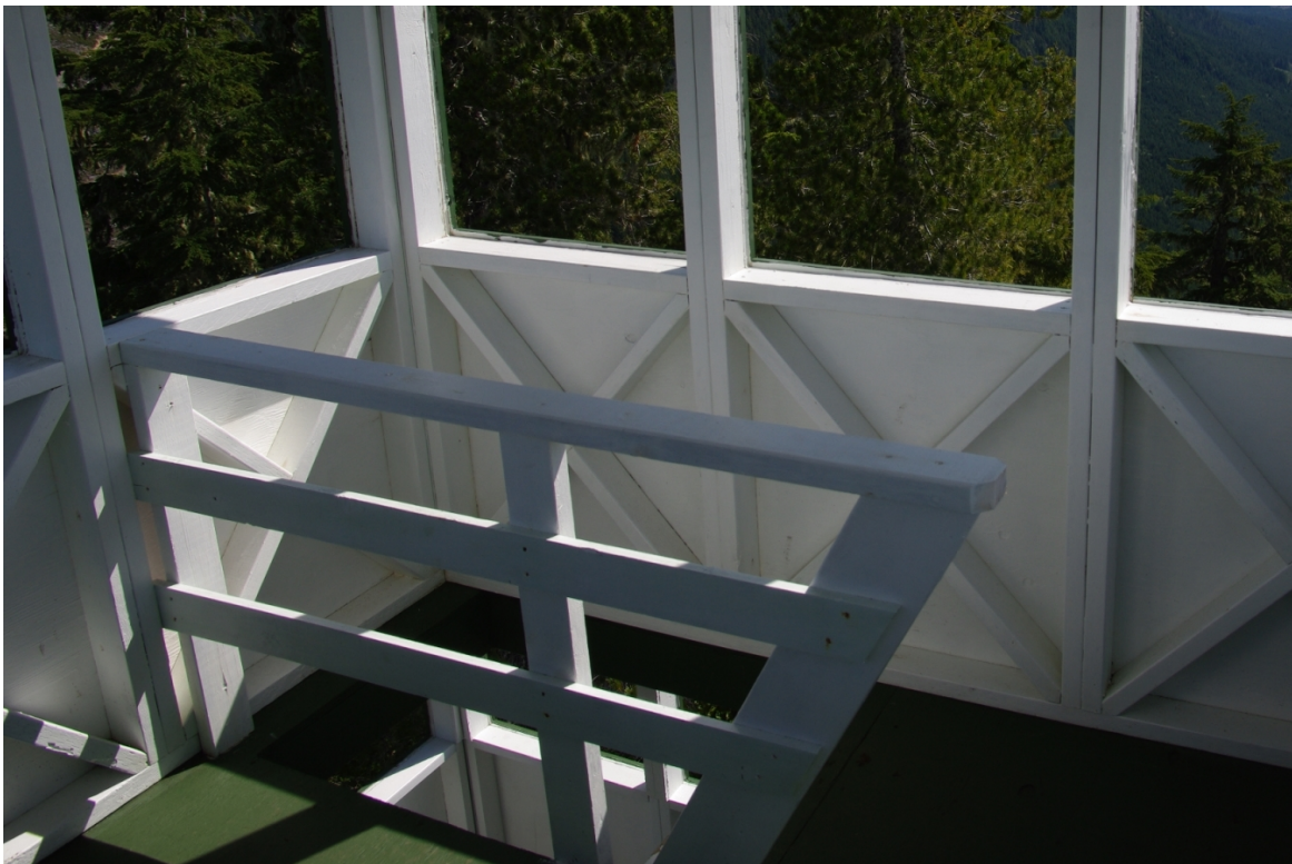
2015: from the cupola looking down through the access opening to the lower level.
