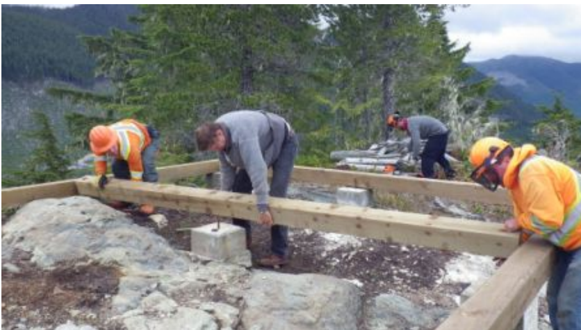
Building the new foundation on the old lookout site
