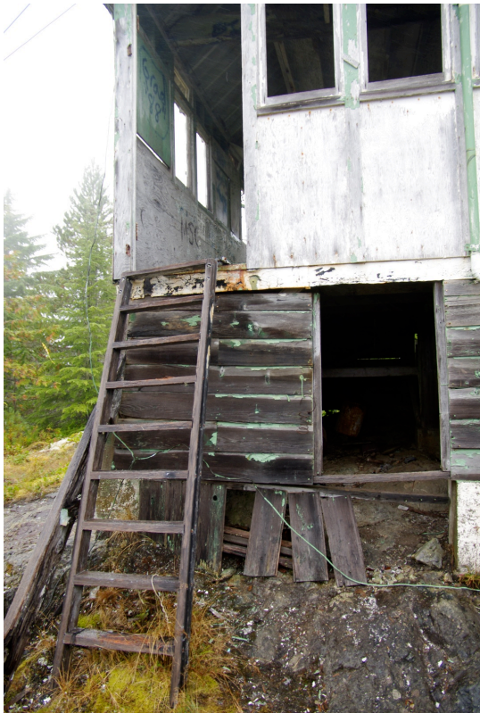
2012: the original entryway faced downslope
