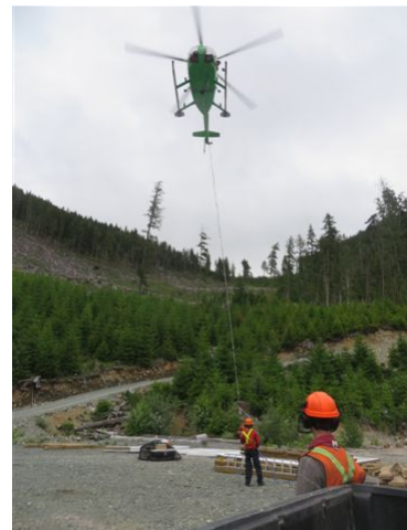
Preparing to transport panel
