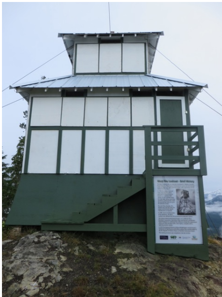
Exterior info sign installed
