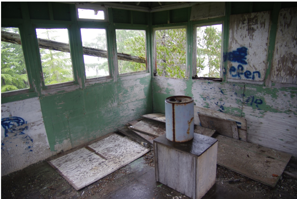
2012: the old fire lookout in disrepair and unsafe; visitors climbed onto bucket and hauled themselves up into the cupola (upper level).
