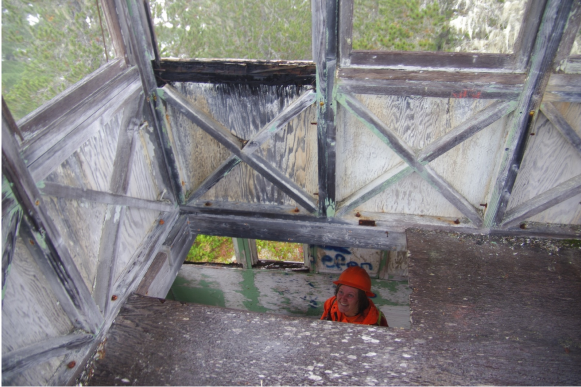
2012: from the cupola looking down through the access opening to the lower level.
