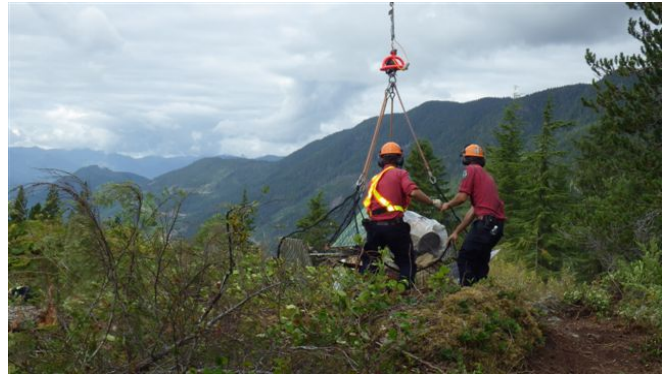
Debris slung out via helicopter
